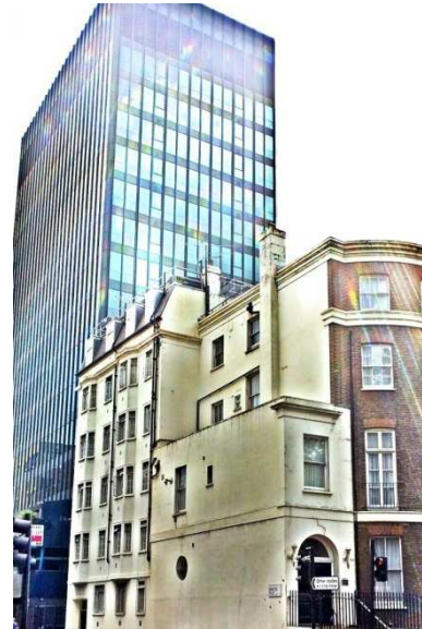
Olallo House TB Hostel
